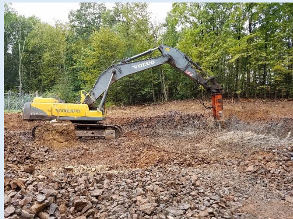
Hoe Ram removing basalt bedrock.
