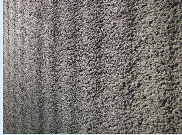
Close-up of tank wall after shotcrete was applied.
