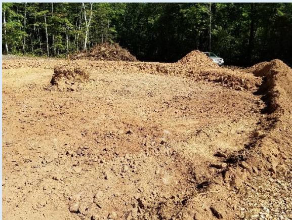
New tank location, topsoil scraped away.
