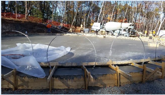
"Seismic" cables will stabilize wall sections.
