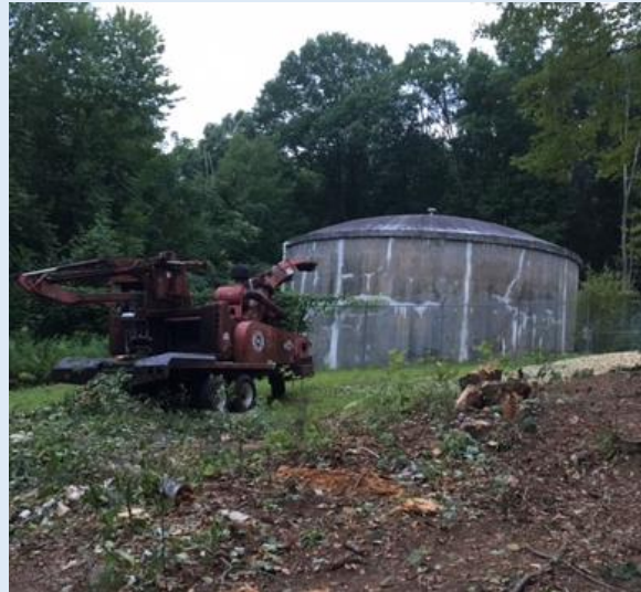
Our present tank, as it looks today.
