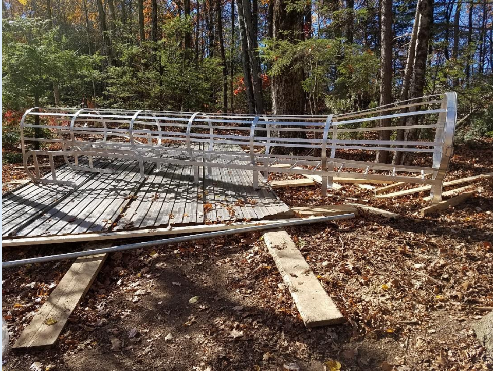
This ladder will provide access to the hatch on the dome, for inspection & testing. A locked plate will prevent unauthorized climbing of the ladder.
