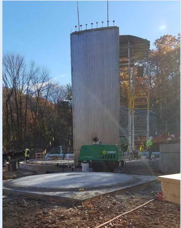
1 st wall panel being lowered onto tank floor.
